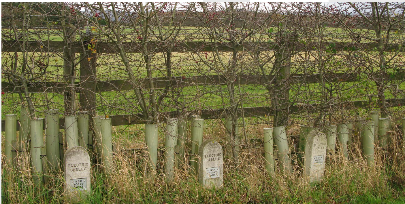
Example of reinstated hedge above underground cables
