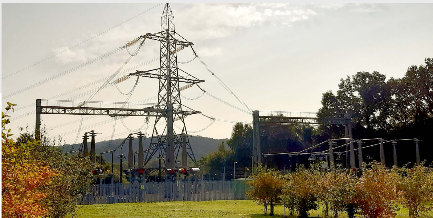
Example of a sealing end compound
